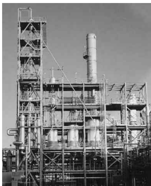
Figure 5.6. Industrial unit using a technology of continuous regeneration of the catalyst (catalytic reforming process by moving radial bed for production of base fuels with a high octane number) © IFPEN
